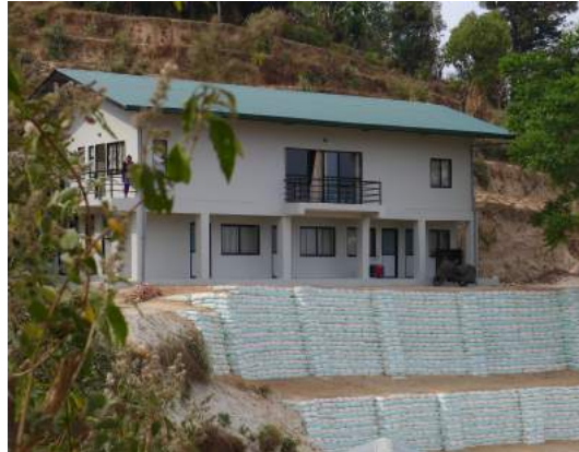
The MMB Centre with its multi-layered wall made out of earthbags
