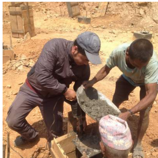
Working on the foundation
